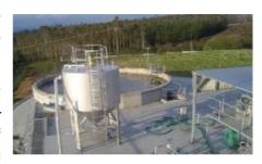
In what concerns the rest of waste-waters of the plant, they are sent to the treatment system. These come exclusively from the washing centre of the lorry exteriors to which later on sanitary waters from toilets and changing rooms are added.
